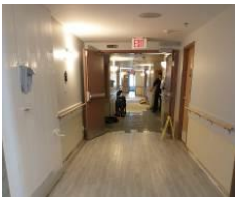
Third Floor Flooring Installation
